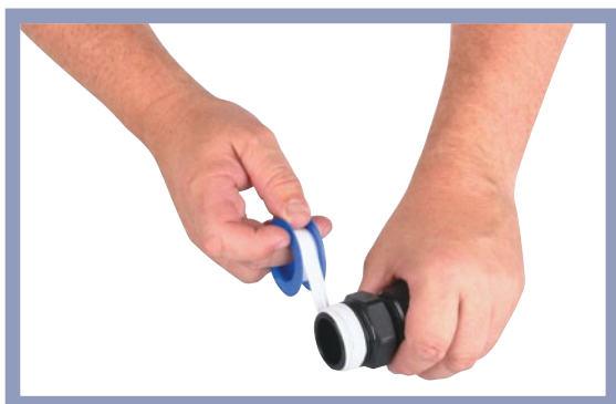
1 (a) Use a teflon tape sealant or
