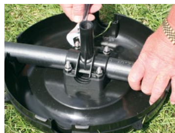
Select the Riser to suit your sprinkler size. Ensure fastening nuts are tightened evenly. Fit O-ring seal to sprinkler riser, locate riser spigot into hole in pipe and fasten the cross tee anchor.
