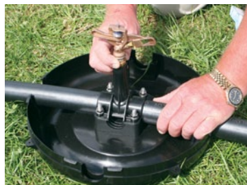
Screw sprinkler into sprinkler riser.
